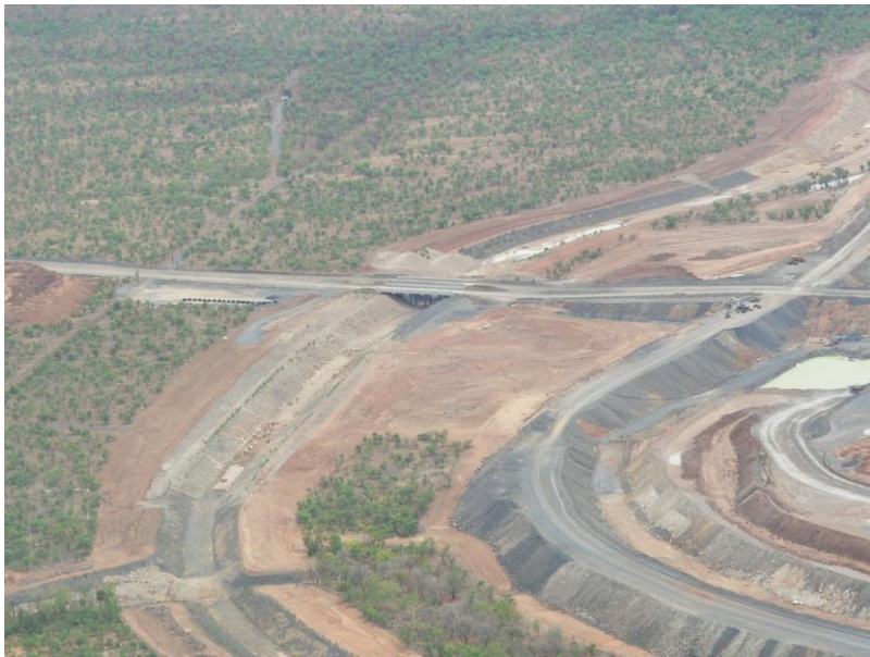
Barney Creek Diversion Channel - 2008
