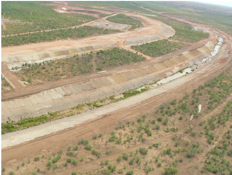
McArthur River Diversion Channel - 2008
