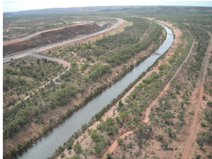
McArthur River Diversion Channel - 2014
