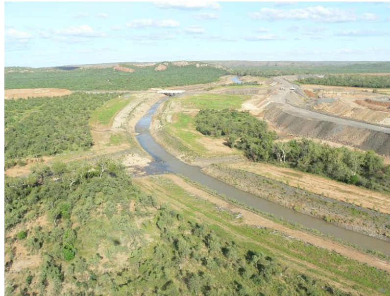
Barney Creek Diversion Channel - 2012
