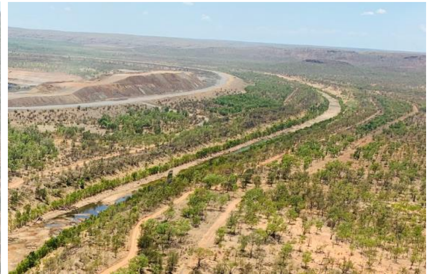
McArthur River Diversion Channel - 2019
