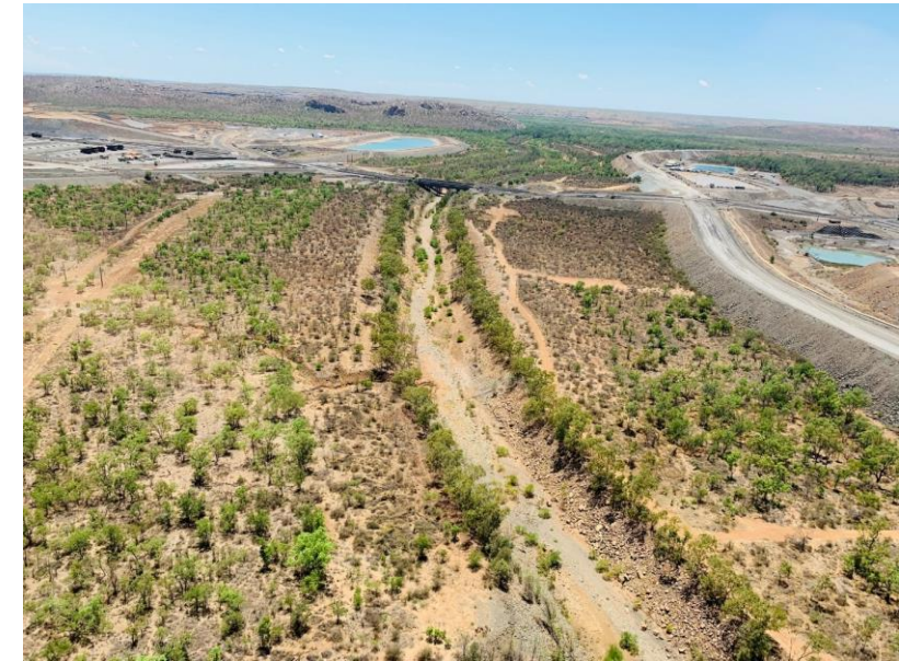
Barney Creek Diversion Channel - 2019
